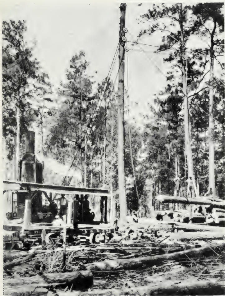
FIG. 50. HIGH LEAD GROUND SKIDDING: HEAD SPAR.
